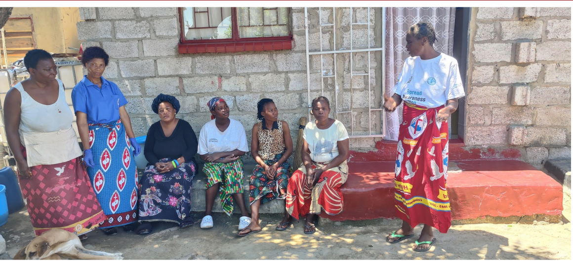
Strengthening IPC in Matero: The Women's Christian Fellowship proudly installs a new tippy tap at their meeting site for United Church of Zambia zonal gatherings Photo Credit:ReAct Africa
